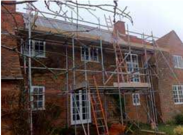
Local scaffold companies x 5
